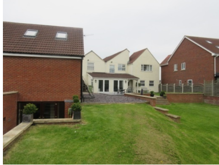
Photo taken facing west towards the rear elevation of No 140
