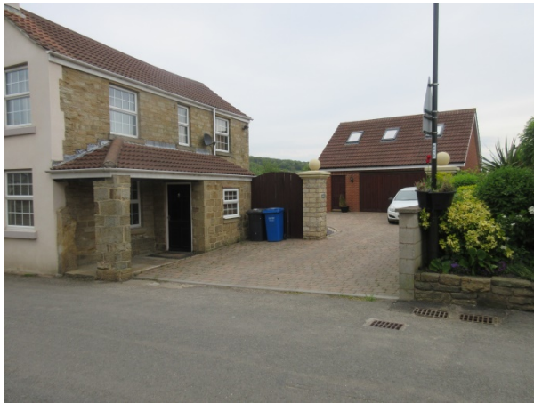
Photo taken from Church Street North highway facing north east
